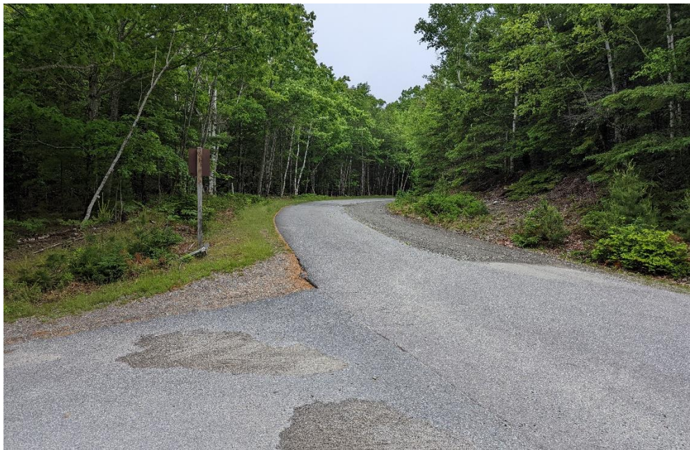
Figure 15 Hulls Cove Visitor Center Potential Bus Charger Area
