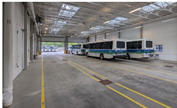
Figure 7 DTI Maintenance Facility Indoor Storage Area
